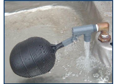
FLOAT & VALVE ASSEMBLY
