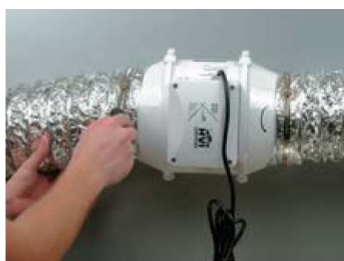
Attach the ducts with clamps.
