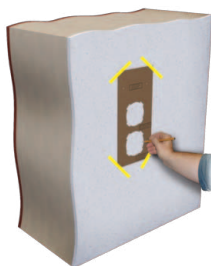
Mark the holes for the air ducts with a cardboard master plate.
