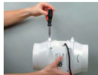
Secure latches by screws.
