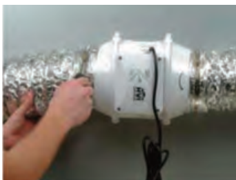
Attach the ducts with clamps.
