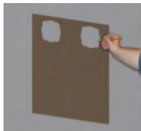
Mark the holes for the air ducts with a cardboard master plate.
