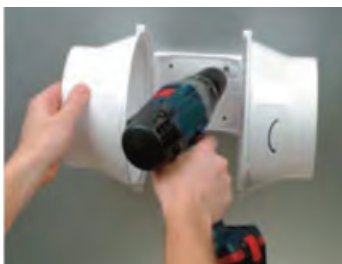
Fix the fan mounting plate on the fl at surface.
