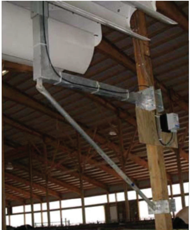
Figure 7 - Cyclone install on a column
